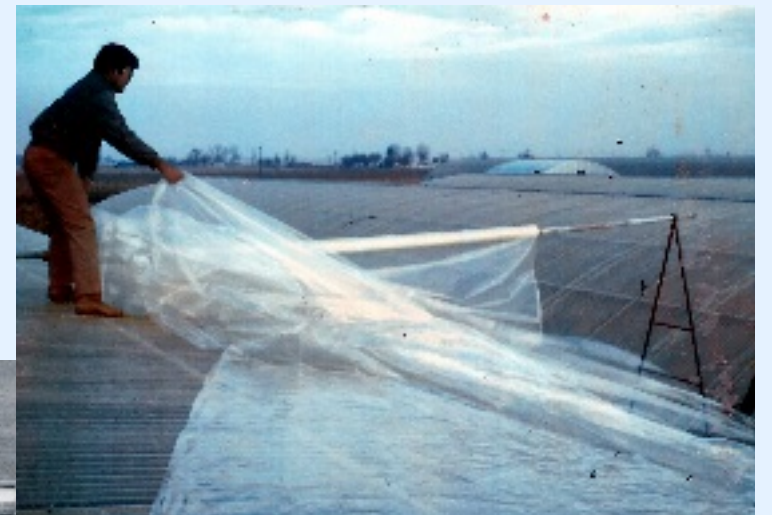
Ken applying polylayer to save heating cost.
