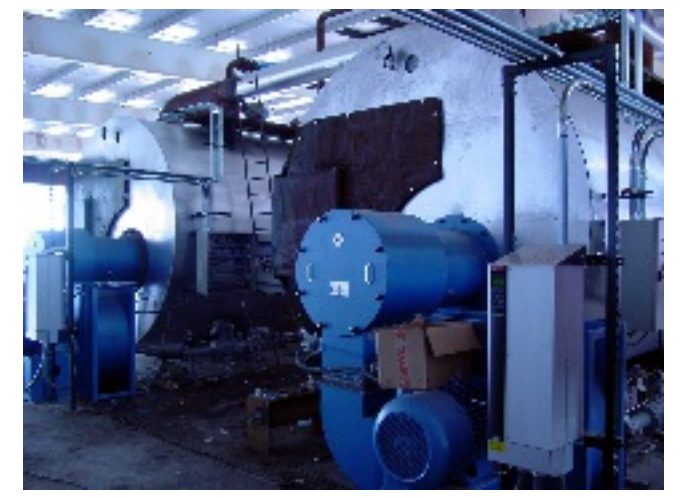
Burners installed on 1000hp boilers
