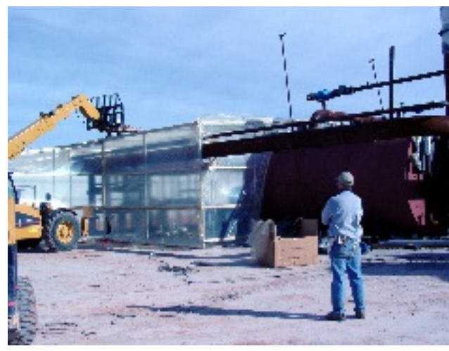
Shelter for boiler plumbing and controls
